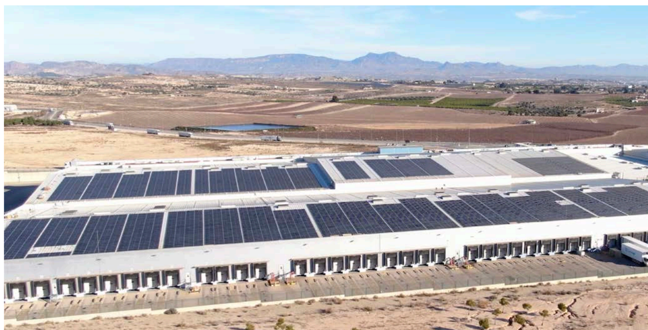
Solar panels at the Las Torres de Cotillas facility (Murcia)
