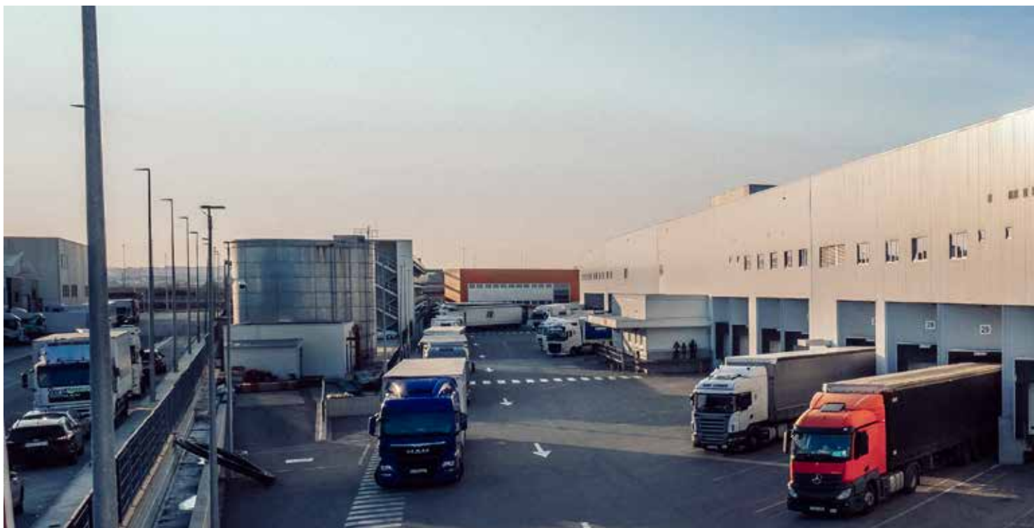
Loading bays at the Silla logistics platform (Valencia)
